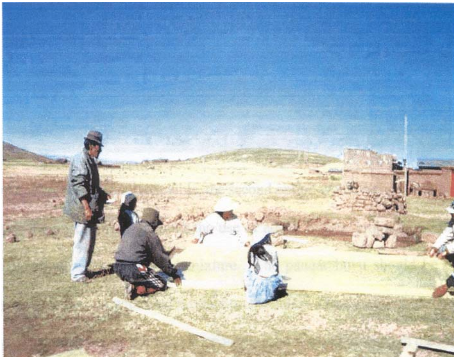
Construction of the covering
